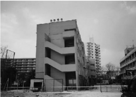
Photo 6.1. Settled school houses in Kobe
