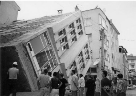
Photo 6.3. A settled building at Site 16 and S4 in Adapazarı
