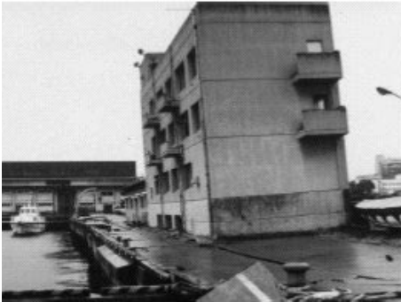
Photo 11.1. Tilted building in lateral spreading area
