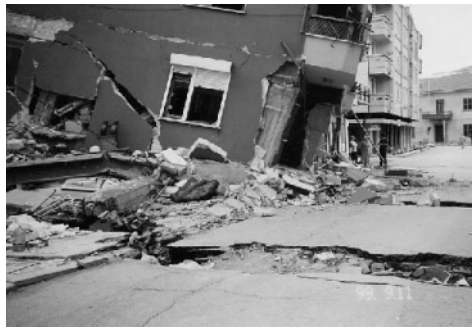
Photo 6.4. A settled building at Site SK4 in Adapazarı
