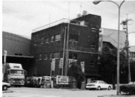
Photo 11.2. Tilted building in liquefied level ground
