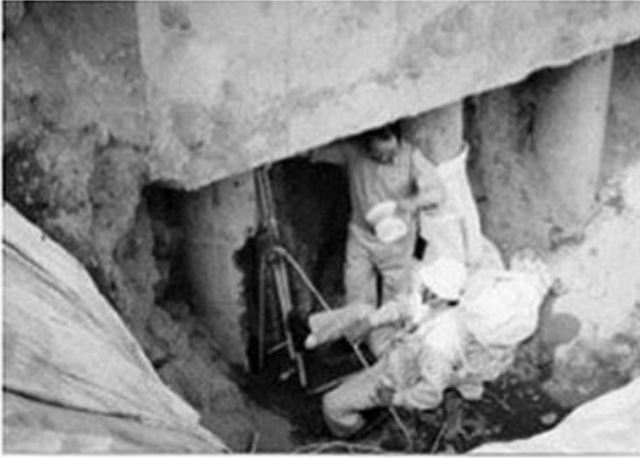
Photo 11.5. Borehole camera survey followed by excavation
